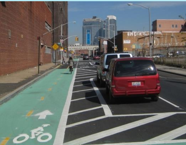
Parking-protected Bike lanes
