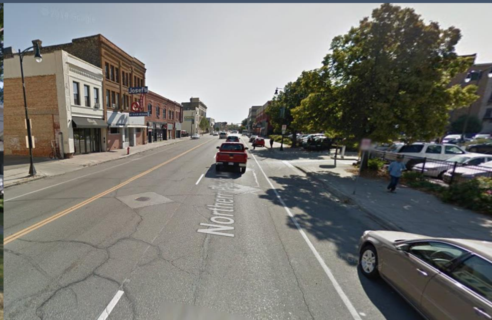
LTS 2: minor arterial with 30 mph speed limit, 3-lanes with on-street parking, some retail
