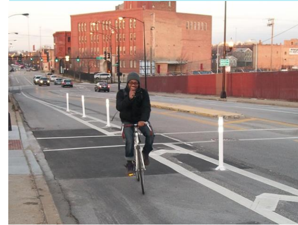
Protected bike lane with flexible bollards
